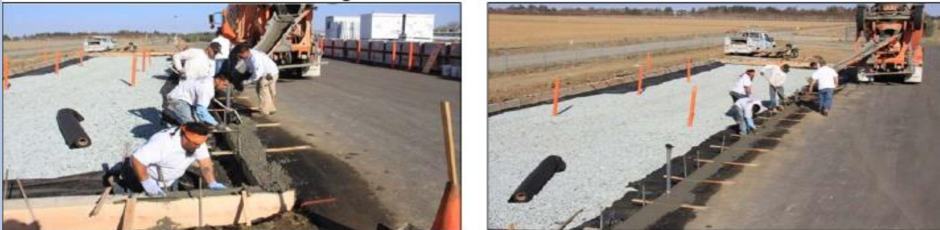
Figure 5.10: Concrete curb placement.
