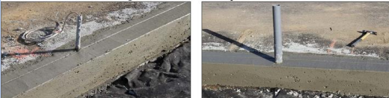
Figure 5.10: Concrete curb placement.
