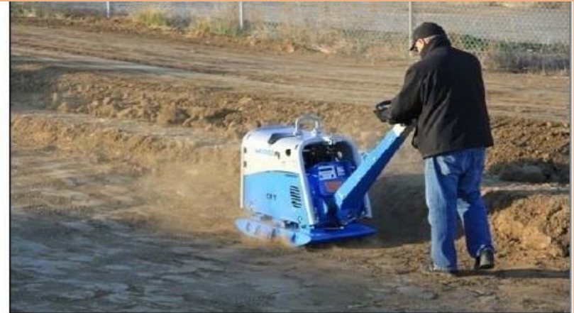
Figure 5.2: Subgrade compaction.
