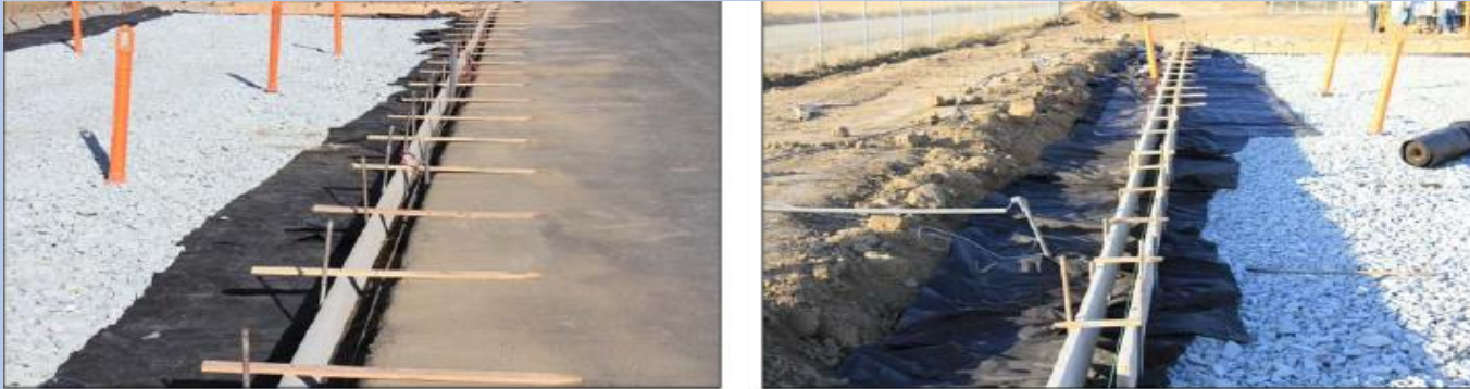
Figure 5.9: Formwork for curb.
