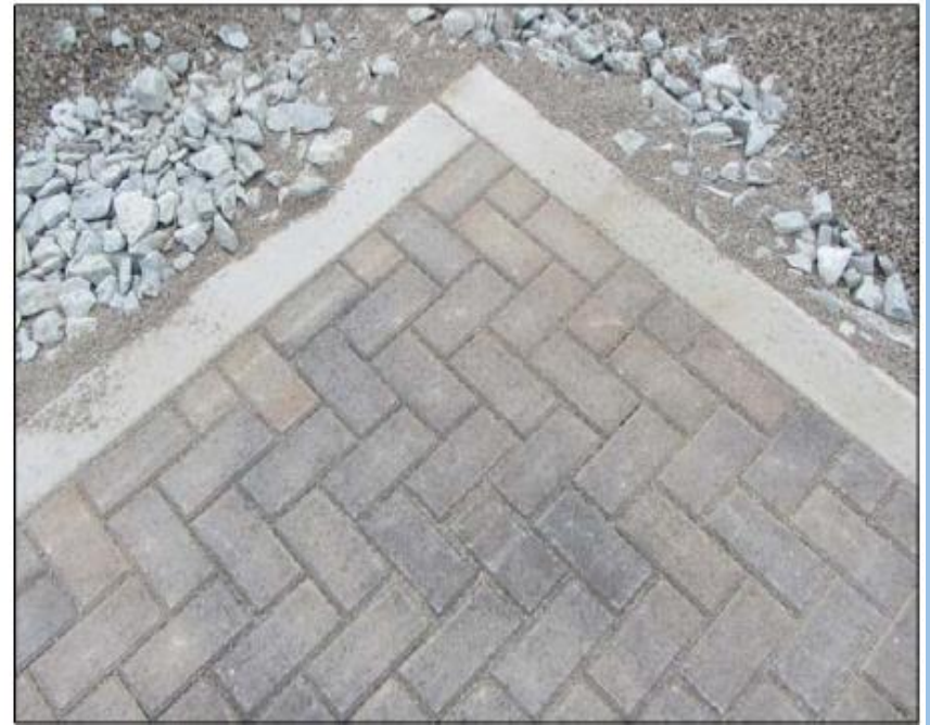
Figure 5.16: Jointing stone placement and compaction.
