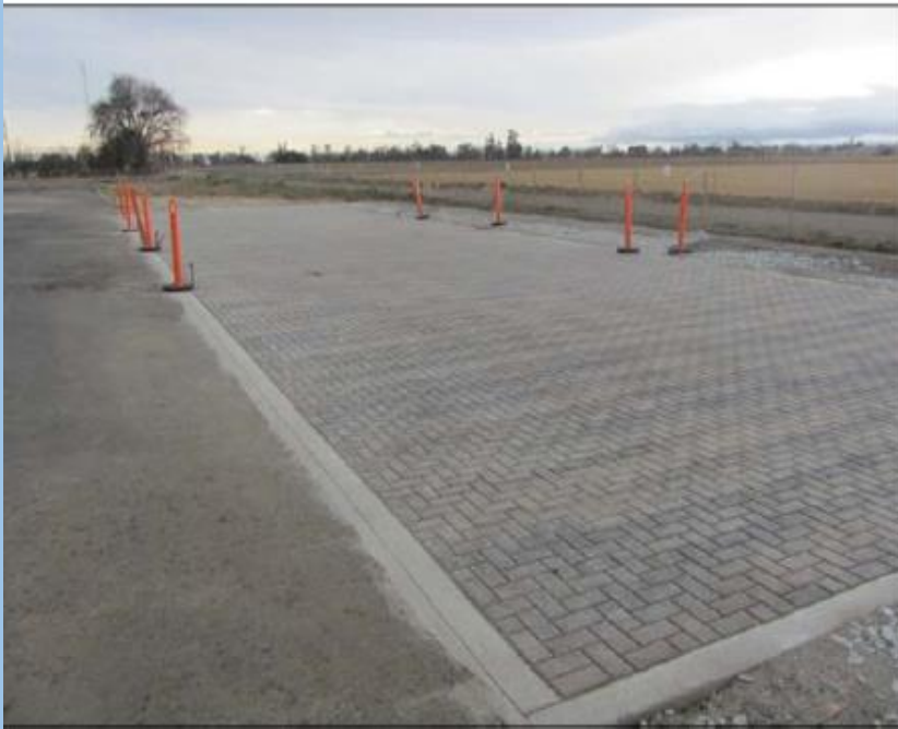
Figure 5.16: Jointing stone placement and compaction.
