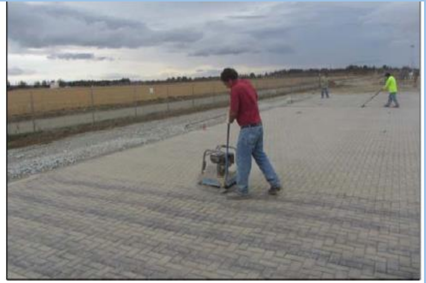
Figure 5.16: Jointing stone placement and compaction.
