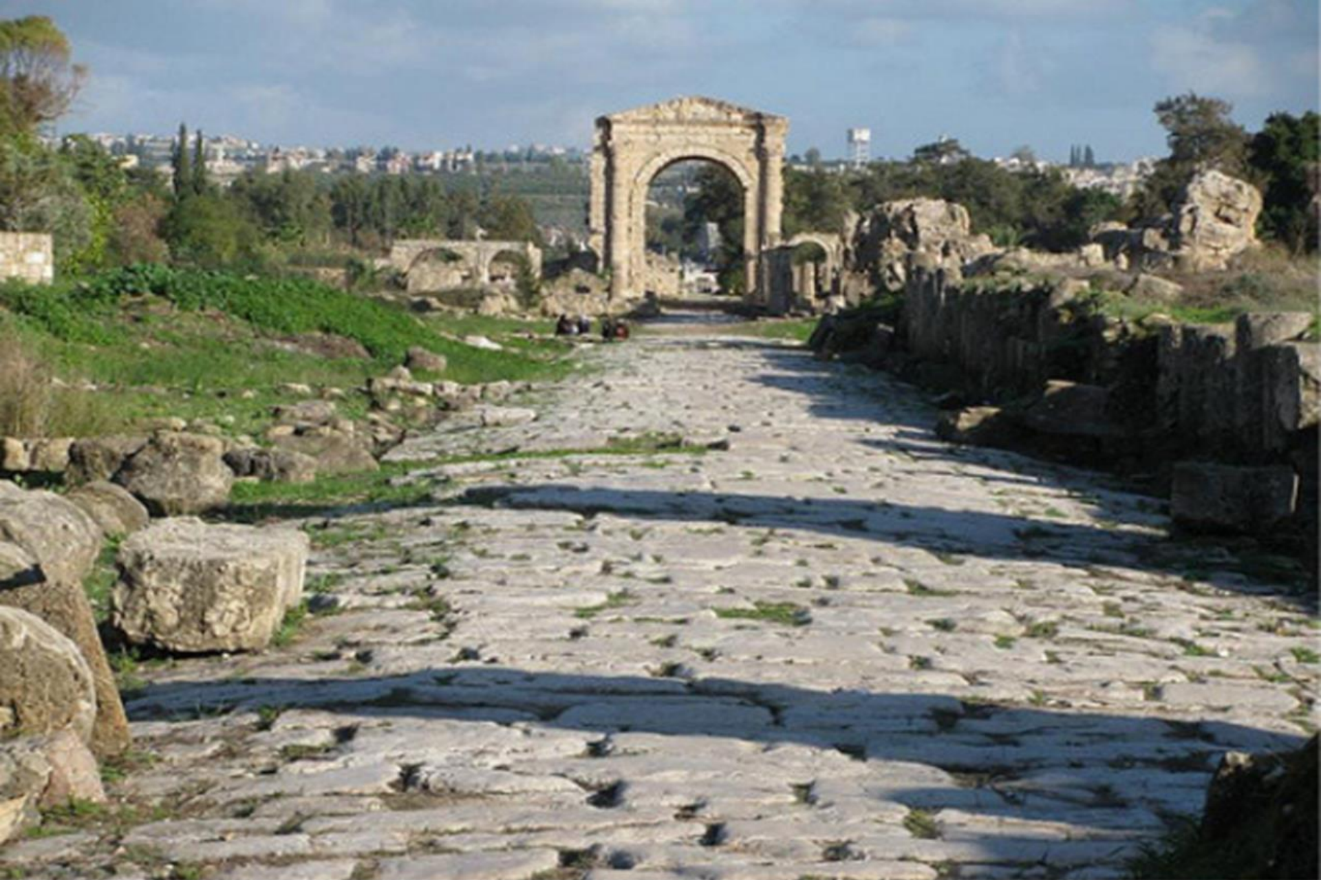
The Appian Way is crowned in middle for storm water flow.
