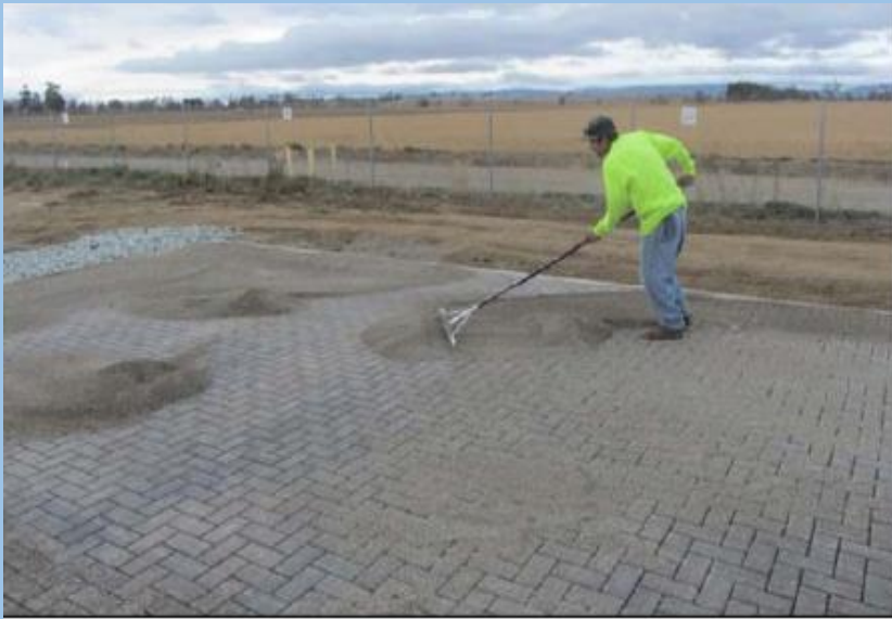
Figure 5.16: Jointing stone placement and compaction.
