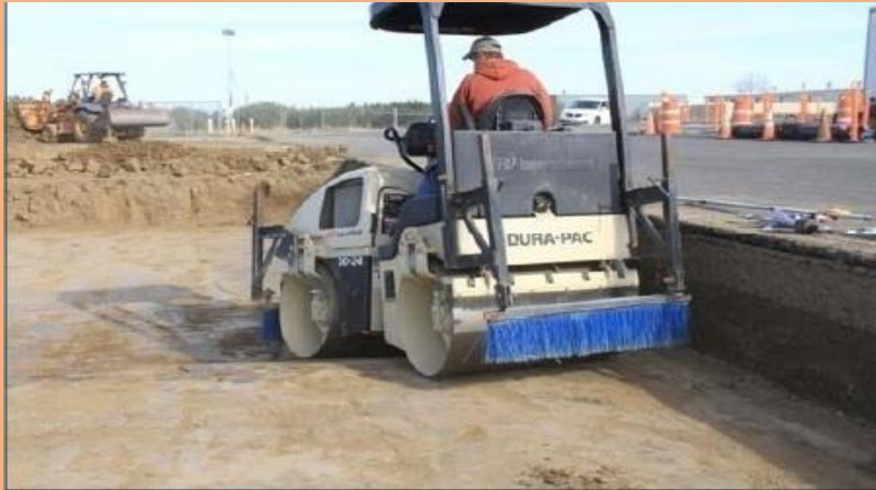
Figure 5.2: Subgrade compaction.
